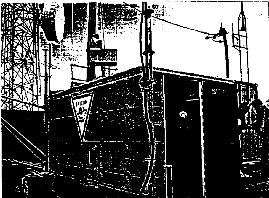
The W6WX/B housing on Mt Umunum. K6GSJ (l) and N6EK (r) are working on some of the coaxial cabling. The GPS unit is mounted on the pole at the far left corner of the housing.
