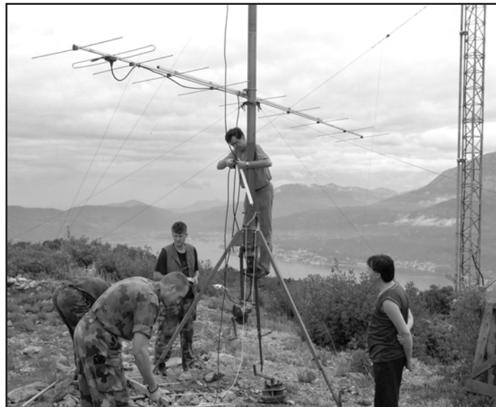
(Left) Pertti, OH2RF, using Armstrong method to rotate 6 Meter beam. (Right) Ranko, YT6A, giving instructions to antenna crew erecting 2 Meter stacked array.
