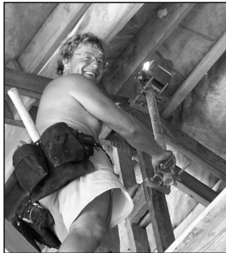
Nature Conservancy employee, Todd Anderson, lends a hand to install the antenna support mount for the warehouse roof antenna.
