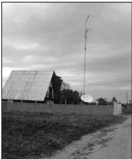
The PW5Q antennas at the PP5RR QTH shows what all WRTC competitors were using. The tower is 17 meters high, topped with an 8-element log periodic and a 2-element 40 Meter Yagi; an 80/75 Meter dipole hangs below the beams. Photo courtesy Ward Silver
