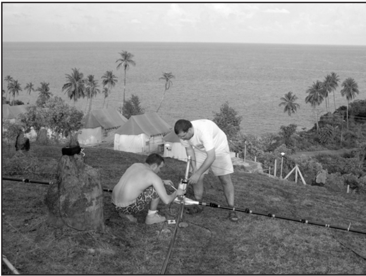
(Left) A view of the camp from the antenna farm while Sylvain Lefevre, F4EGD, and Flo Moudar, F5CWU, assemble one of two Spider beams. (Right) Preparing the mast for raising the 5-band Spider beam.
