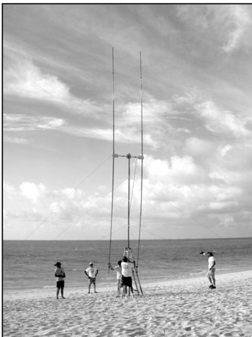
Erecting the 2-element SteppIR antenna.
