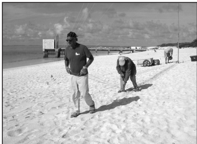
We needed to bury the ground radials to prevent seals from becoming entangled in them.
