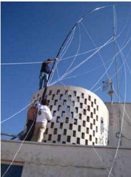
David Jorgensen, WD5COV, Franz Langner, DJ9ZB, and Kazu Fujita, JH1OGX, wrestle our 160 Meter vertical to the roof.
