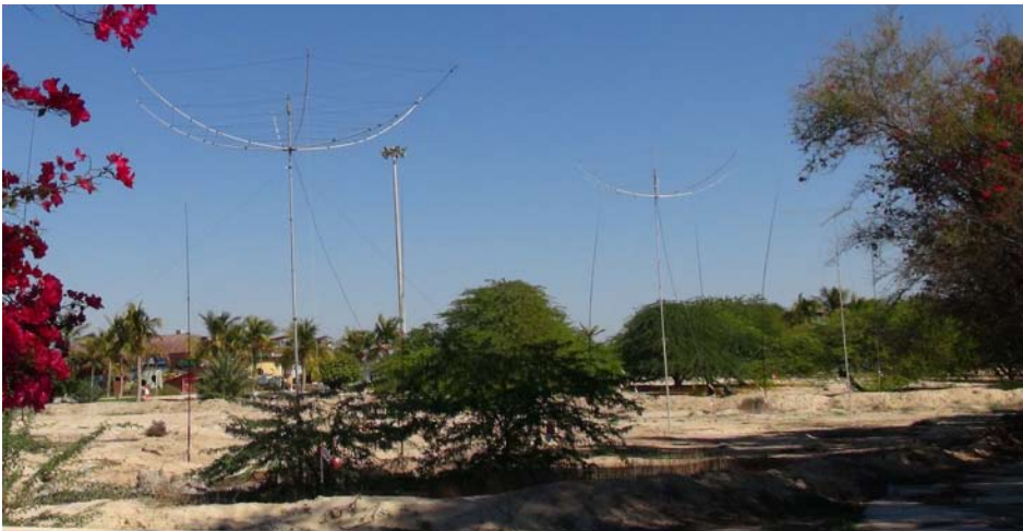
The antennas: 80M vertical, phased array 30M, HexBeam 15-20, HexBeam 17, 4-square 40M and beam 10M.
